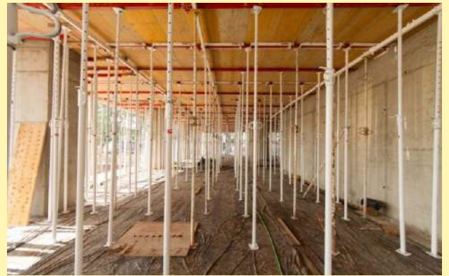
BACK - PROPPING THE SLAB
