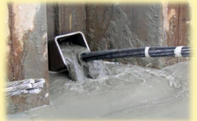
GROUTING OF ANCHORS
