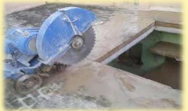
SLAB CUTTING WORK
