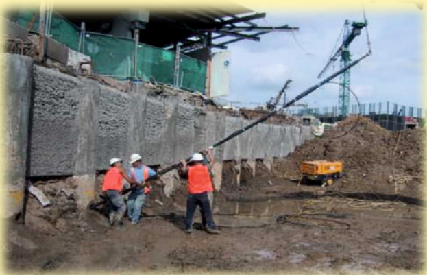
INSTALLATION OF ANCHOR
