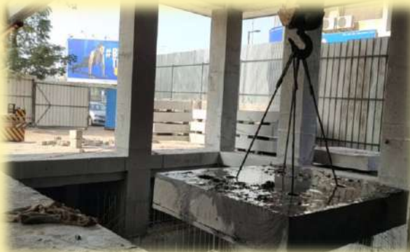
CUTTING PIECE SHIFTING
