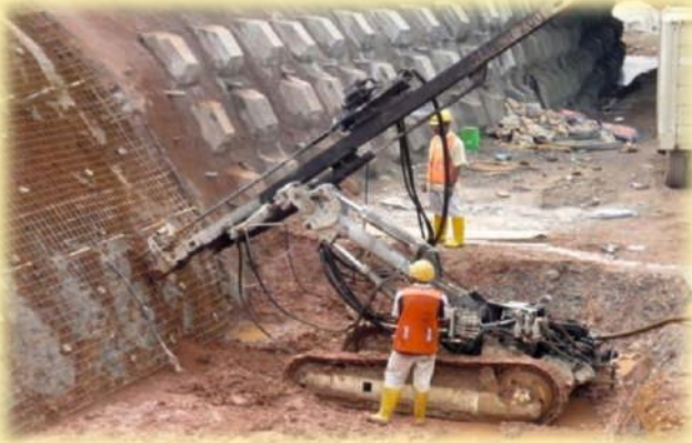
DRILLING OF BORE HOLES
