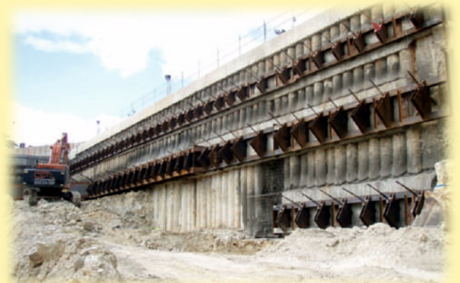
INSTALLATION OF WALLER BEAMS
