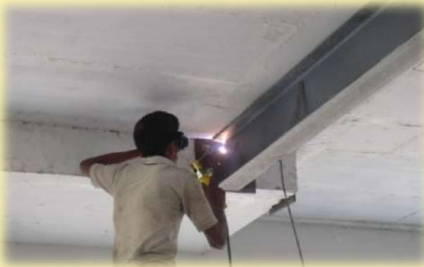
ISMB/ ISMC STRENGTHENING
