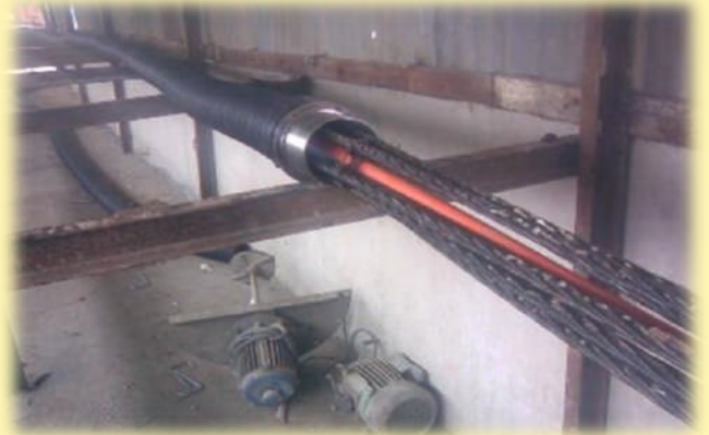
FABRICATION OF ANCHORS
