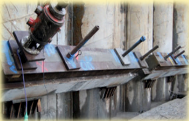
STRESSING OF ANCHORS
